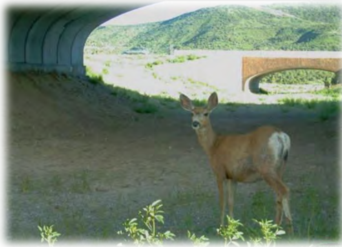
Figure D-19. Mule deer used the arch underpass under I-70 in Utah. Photo Credit: P. Cramer, Utah Department of Transportation, and Utah Division of Wildlife Resources.
