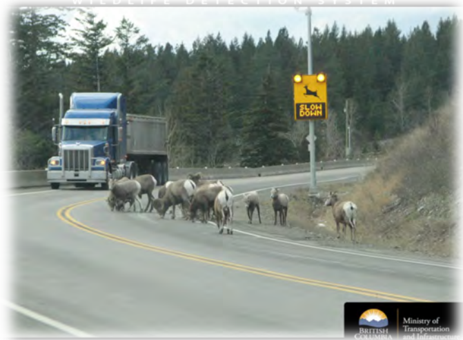
Figure D-55. British Columbia Ministry of Transportation and Infrastructure installed a radar based animal detection driver warning system on Highway 3. Photo Credit, British Columbia Ministry of Transportation and Infrastructure.
