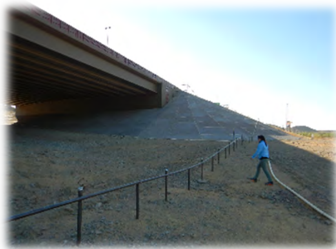
Figure D-30. Arizona placed a steel rail fence at a wildlife underpass structure to deter motorized vehicle use. Photo Credit: Arizona Game and Fish Department.
