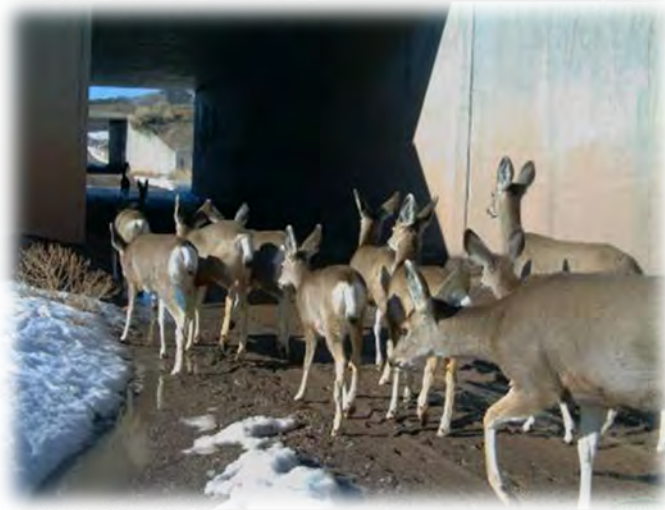
Figure D-22. In Utah, once wildlife exclusion fence was placed along this USDA Forest Service road that encompassed a pair of concrete box culverts, mule deer began using these to pass beneath Interstate 70, with hundreds of successful mule deer movements through the pair of culverts each year (Cramer 2012, 2014). Photo Credit: P. Cramer, Utah Department of Transportation, Utah Division of Wildlife Resources.
