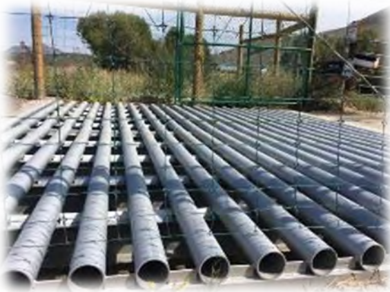
Figure D-44. Left, Colorado SH 9 round bar double cattle guard. Photo Credit: P. Cramer. Photo on right demonstrates how mule deer can use the support beams to breach the guard. Photo Credit: Colorado Department of Transportation, Colorado Department of Parks and Wildlife, and ECO-resolutions.
