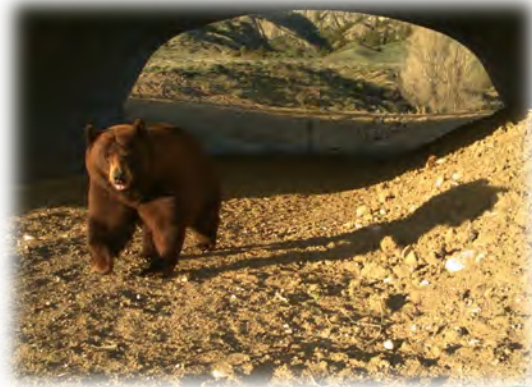
Figure 3-11. Colorado’s State Highway (SH) 9 Wildlife Mitigation Project was planned for and funded because of safety concerns for motorists, wildlife safety and connectivity, and committed partners with Colorado DOT. Black bear used this and most underpasses in the project. Photo Credit: Colorado DOT, Colorado Fish, Wildlife, and Parks, and ECO-resolutions. See this project in Appendix A. Case Studies .
