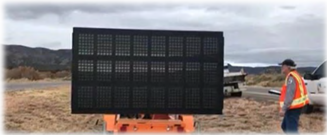
Figure D-52. M. Watson of New Mexico Department of Game and Fish installed driver warning variable message board with New Mexico Department of Transportation maintenance personnel. Photo Credit: New Mexico Department of Game and Fish.
