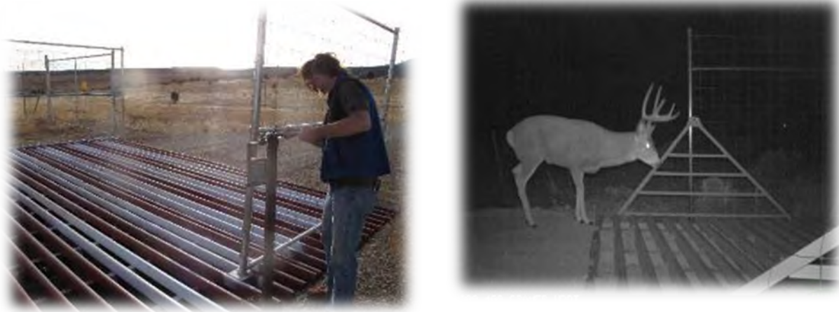
Figure D-40. Left, Utah's double cattle guards with appropriate side fences and aprons, no mid-guard support, and rounded top bars of a guard. Photo Credit: P. Cramer. Mule deer ponders a flat bar Utah double cattle guard on US 89 and was deterred. Photo Credit: P. Cramer, Utah Department of Transportation, and Utah Division of Wildlife Resources.
