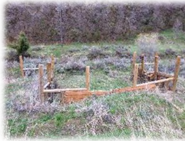
Figure D-37. A Utah high migration escape ramp on US 91. Three sides provide three escape opportunities. Photo Credit: P. Cramer. Photo on Right, Mule deer uses a high migration escape ramp in Utah, US 91. Photo Credit: P. Cramer, Utah DOT, Utah Division of Wildlife Resources.
