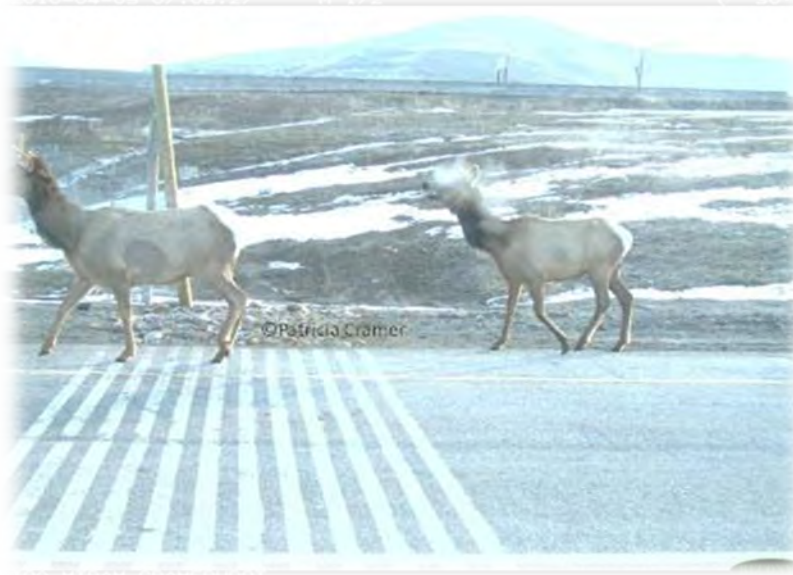
Figure D-49. Elk move over painted lines mimicking cattle guard in Utah along Interstate 80. Photo Credit: P. Cramer, Utah Department of Transportation, Utah Division of Wildlife Resources.
