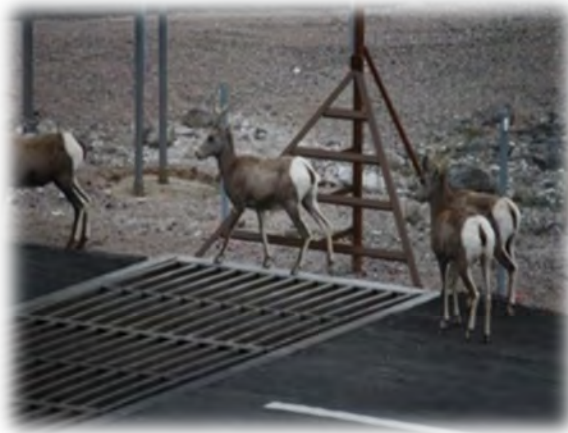
Figure D-43. Left, desert bighorn sheep breach a single cattle guard by using support lip in Arizona. Right, the guard was adapted to a double cattle guard and the vault lip was covered with fence. Monitoring found no bighorn breaches after retrofit. Photo Credit: Arizona Game and Fish Department, Arizona DOT.
