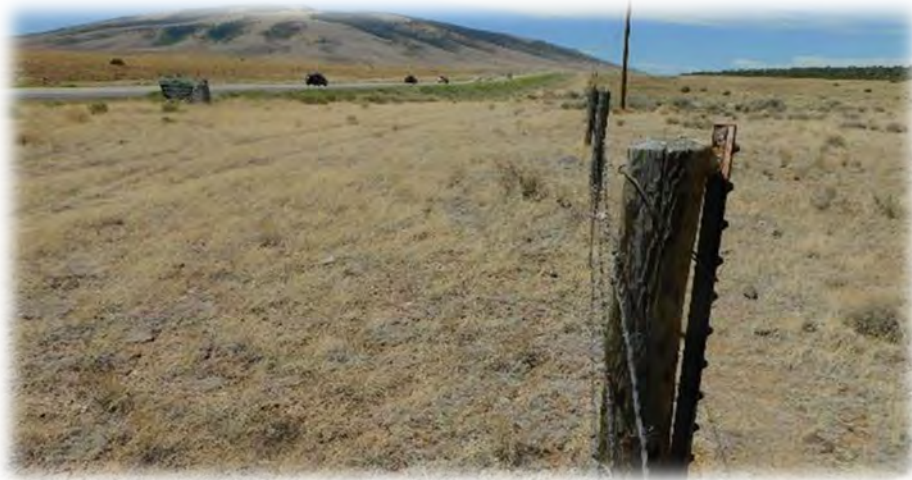
Figure D-8. Lay-down fence in erect setting with permanent metal posts supporting wooden lay-down posts, on the Rio Grande Del Norte National Monument, Tres Piedras, New Mexico. Photo Credit: P. Cramer.
