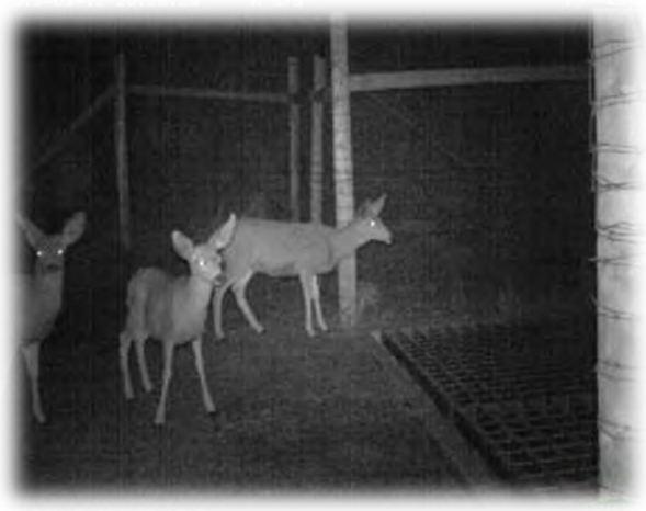
Figure D-42. Left, a wildlife guard in Utah, on US 91. Mule deer breached the guard by walking on the outer lip of the vault. Photo Credits: P. Cramer, Utah Division of Wildlife Resources.
