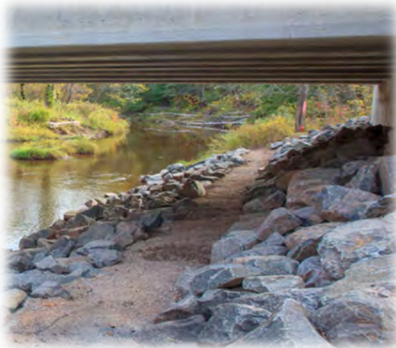
Figure D-4. Minnesota passage bench (left) and aggregate surfacing (right) to treat rip rap to provide soil structure for wildlife and human passage. Photo Credits: Minnesota Department of Natural Resources, courtesy of P. Leete.
