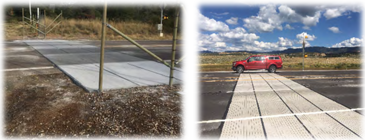
Figure D-47. Electrified barriers installed along SR 260 in Arizona (left), and in New Mexico (right) along US 550 to keep elk and deer out of the fenced right-of-way. Photo Credit: Arizona Game and Fish Department.
