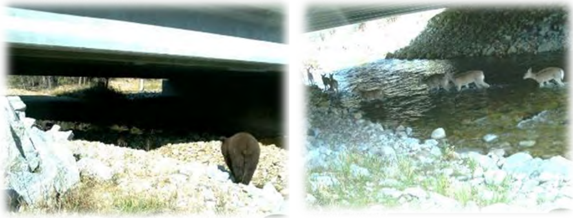
Figure D-16. In Montana, black bear and white-tailed deer used bridged wildlife crossing structures with water features. Photo Credit: P. Cramer and Montana Department of Transportation.
