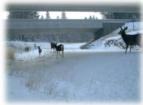
Figure 2-4. Mule deer move beneath US 97 in the Lava Butte Wildlife Mitigation Project area, south of Bend, Oregon. Wildlife-friendly crossing structures were placed in the road widening project. Photo Credits; Oregon DOT, Portland State University, P. Cramer.
