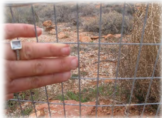
Figure D-32. Types of fences and wall to keep amphibians, reptiles, and small animals off the road and moving toward wildlife crossings. Top, Paynes Prairie Preserve, Florida, concrete wall for reptiles and amphibians prior to construction completion in 1999, Photo Credit, P. Cramer; Middle, chain link fence for turtles, in Minnesota, Photo Credit, C. Smith, Minnesota DOT; Bottom, small grid metal fence to guide tortoises to crossing structures in southern Utah, Photo Credit, P. Cramer.
