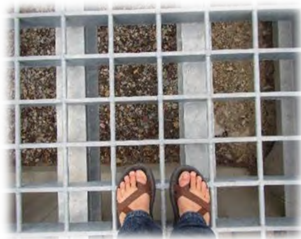
Figure D-42. Left, a wildlife guard in Utah, on US 91. Mule deer breached the guard by walking on the outer lip of the vault. Photo Credits: P. Cramer, Utah Division of Wildlife Resources.
