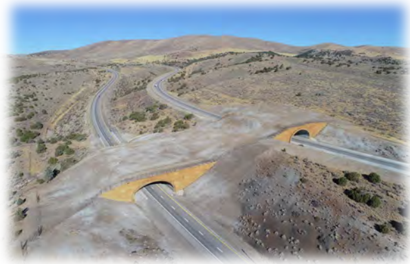
Figure 3-22. Nevada DOT built a set of wildlife overpasses over Interstate 80 on the Pequop Summit ridge line to accommodate migrating mule deer, elk, and pronghorn. Photo Credit: Nevada DOT.
