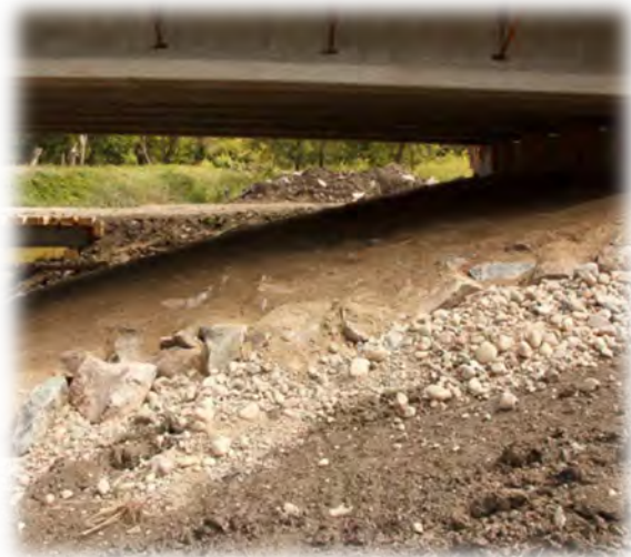
Figure D-4. Minnesota passage bench (left) and aggregate surfacing (right) to treat rip rap to provide soil structure for wildlife and human passage. Photo Credits: Minnesota Department of Natural Resources, courtesy of P. Leete.
