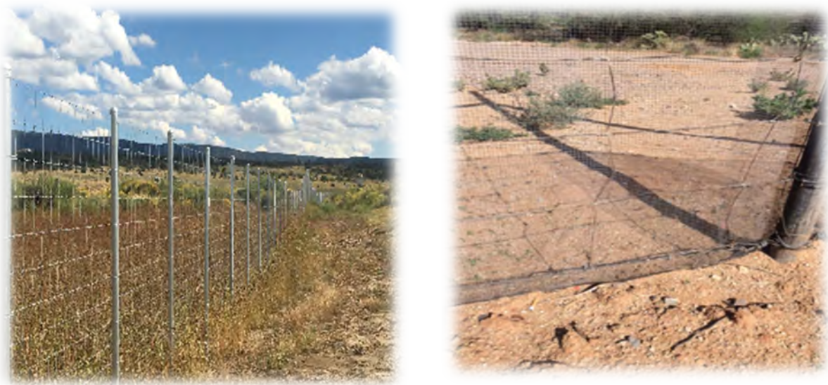
Figure D-28. Fence types: left – traditional right-of-way fence eight feet (2.4 meters) high, right – woven wire mesh fence for smaller wildlife. Photo Credits: Arizona Game and Fish Department.
