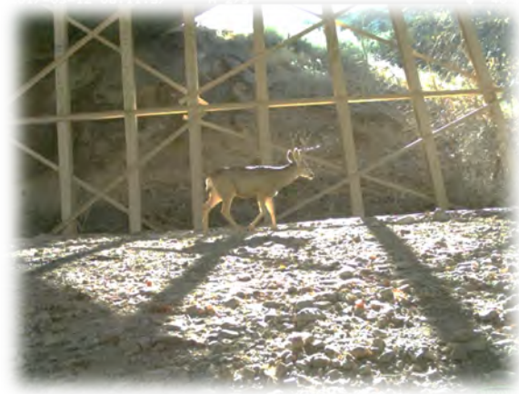
Figure E-14. Example from New Mexico monitoring of smaller culvert where capturing both approaches and crossings of deer and other wildlife was beneficial to furthering knowledge of the success of mitigation measures (left); and a larger structure that will generally pass most local species.
