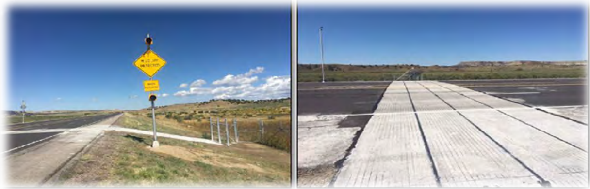
Figure D-60. Driver warning signs and electrified barrier at fence end on US 550, New Mexico. Photo Credit: Arizona Game and Fish Department.
