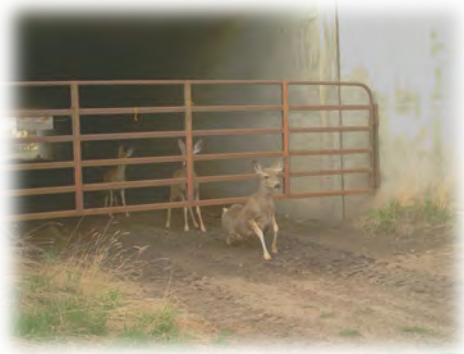
Figure 3-19. In Idaho, monitoring culverts documented the need for Idaho Transportation Department (ITD) to work with adjacent landowners to pull private gates off of the ITD culvert to facilitate wildlife connectivity under Interstate 84. Photo Credit: P. Cramer, M. Schwender, and Idaho Game and Fish.
