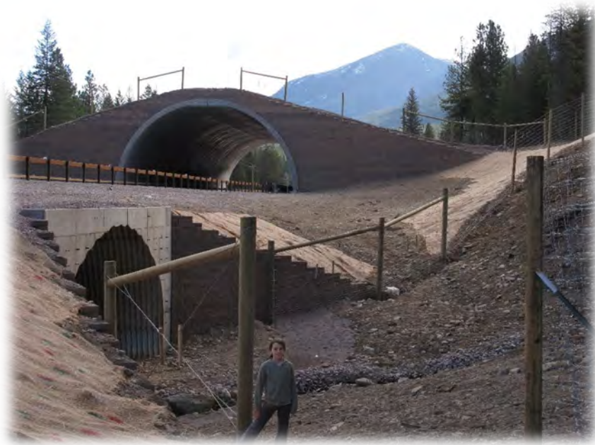
Figure D-9. Montana’s US 93 wildlife overpass, a wildlife underpass, and wildlife exclusion fence. Photo Credit: P. Cramer.
