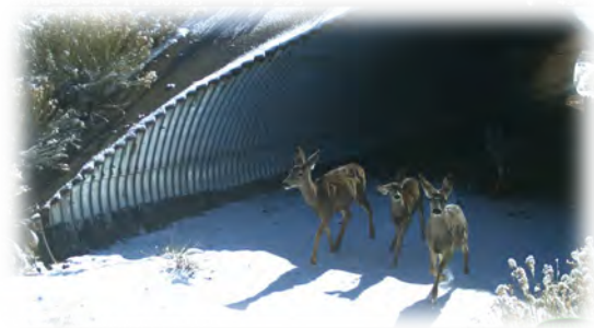
Figure 3-13. The Bureau of Land Management secured over one million dollars in federal funding for wildlife crossing structures on US 89 across the Grand Staircase Escalante National Monument in Utah. Photo Credit: P. Cramer, Utah DOT, and Utah Division of Wildlife Resources.
